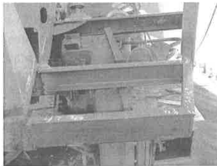
New channel iron framing installed.
