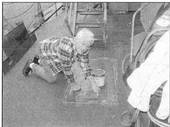
Jim applying a coat of primer.
