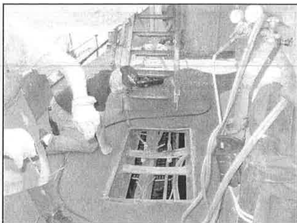
Jim Sr. looking over area that was cut out.
