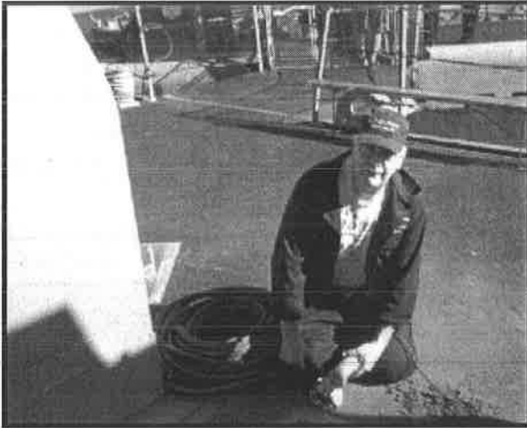
John removing paint in preparation for cutting deck section out.
