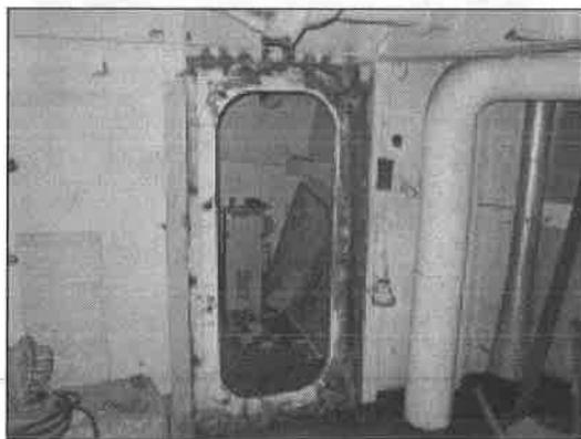
Watertight door frame, tack welded in place.
