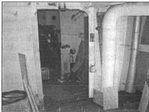
Opening in bulkhead before door frame was set in place.
